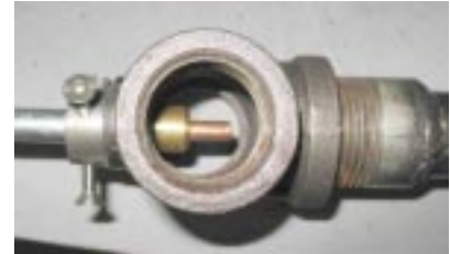
Figure 15: A “T” burner with tip 1” from junction
